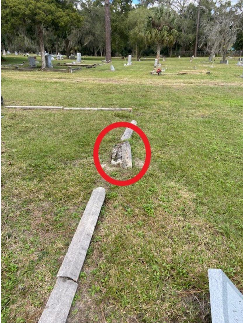
*Attachment 1. An example of damaged and hazardous coping (circled).*
