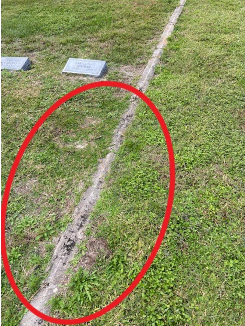
*Attachment 2. An example of damaged and hazardous coping (circled).*
