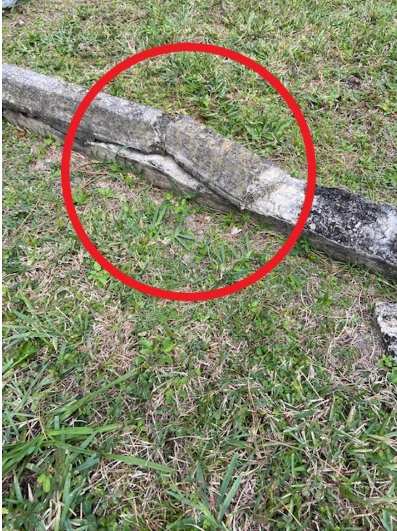
*Attachment 3. An example of damaged and hazardous coping (circled).*
